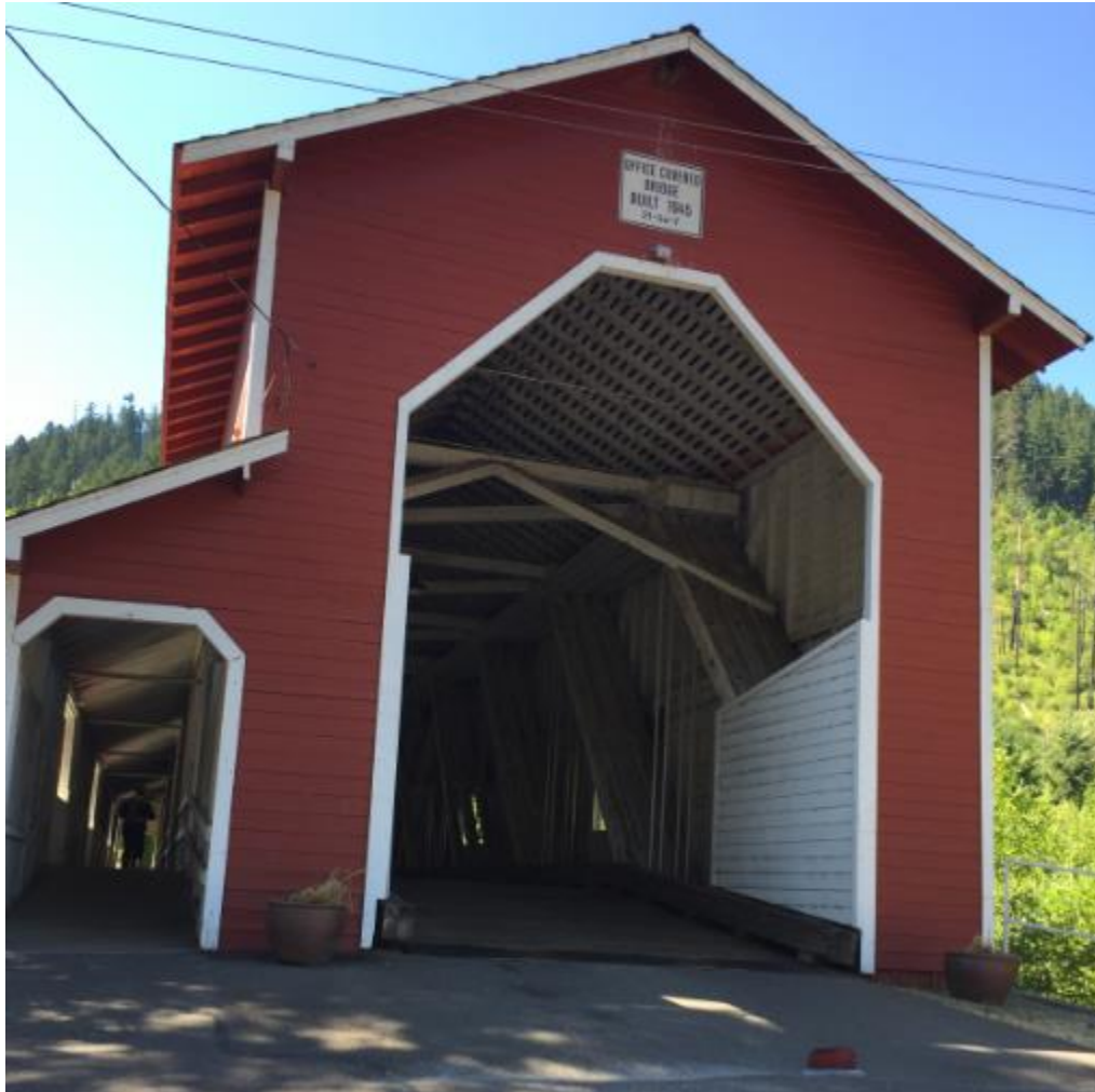
Wood bridge in Oregon.
